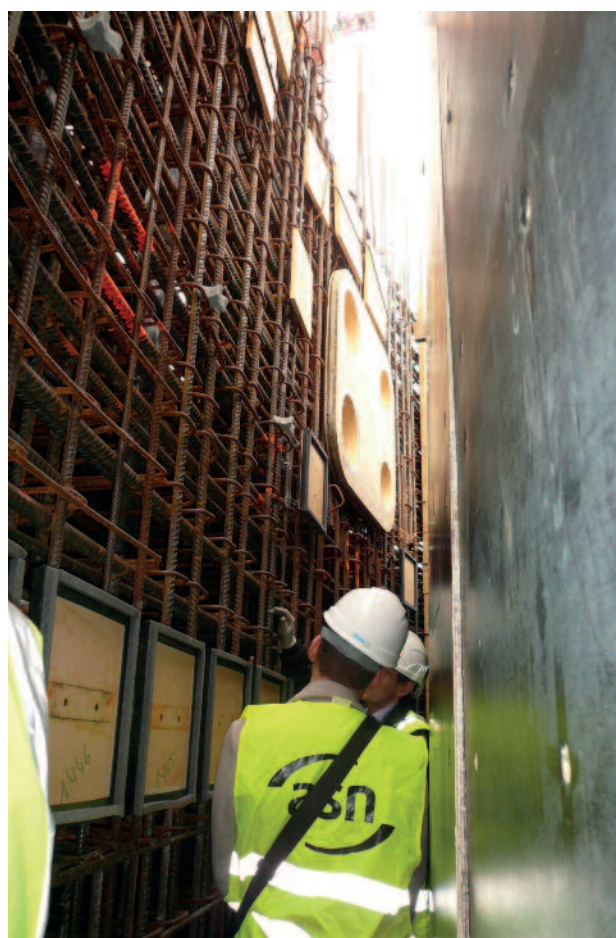
ASN inspection of the reinforcing of the JHR containment – December 2011
