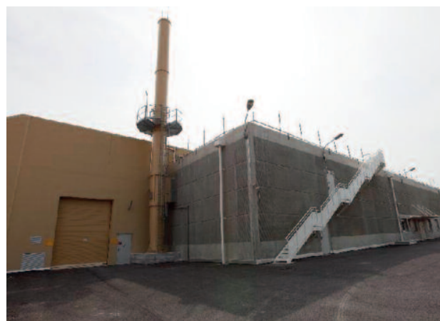
View of the MAGENTA facility at Cadarache
