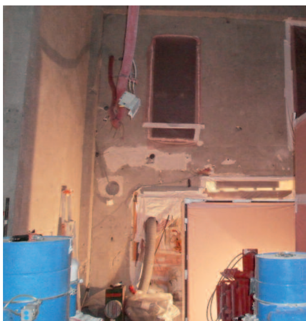
Clean-out work in the “U02 building” before dismantling
