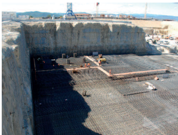
ASN inspection on the ITER construction site – July 2011
